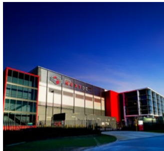
P1 Perth 4 Millrose Drive, Malaga WA 6090
