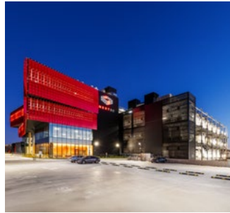
M2 Melbourne 75 Sharps Road, Tullamarine VIC 3043
